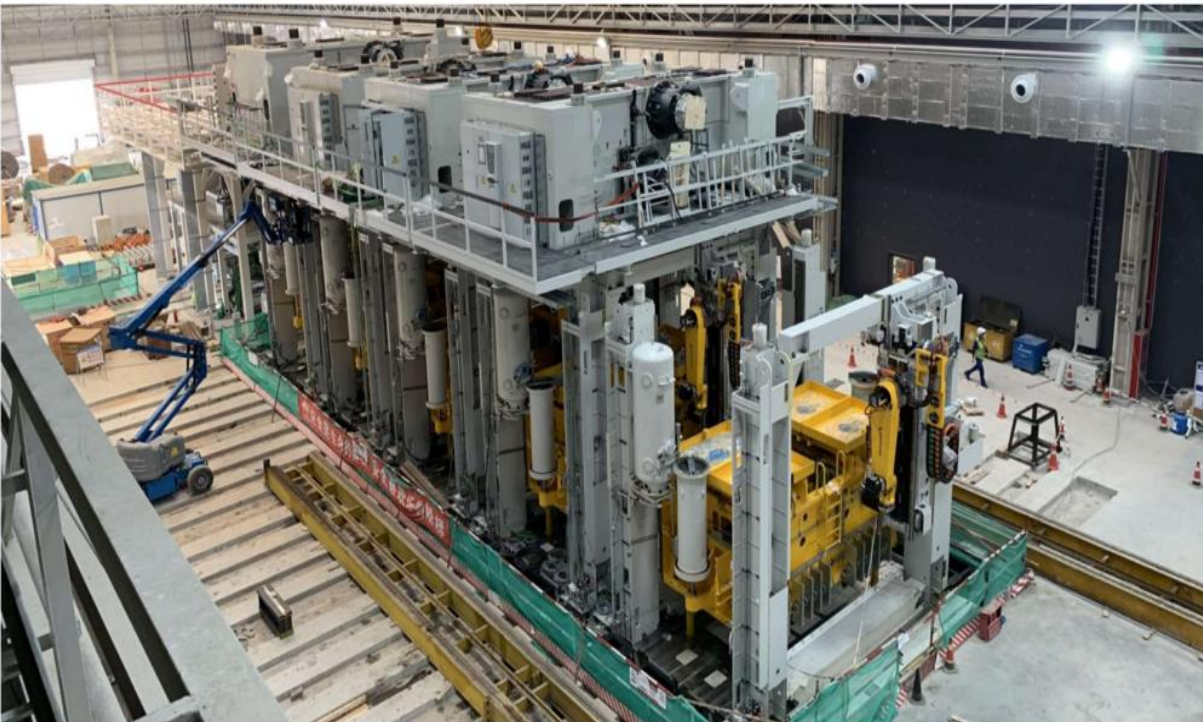
GIGAFACTORY SHANGHAI - MODEL Y FACTORY INTERIOR
